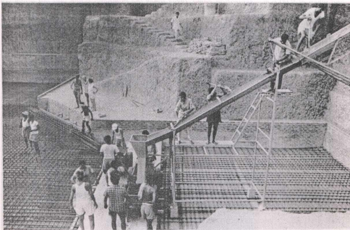
Starting to pour the concrete of the 22cm thick tie-slab
